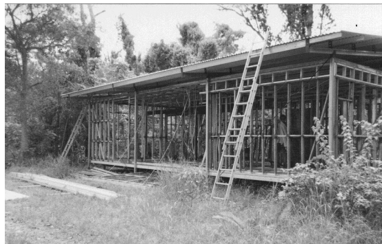
The Caretaker's Cottage Building at Riyala. At this stage part of the wall frame is still missing.
