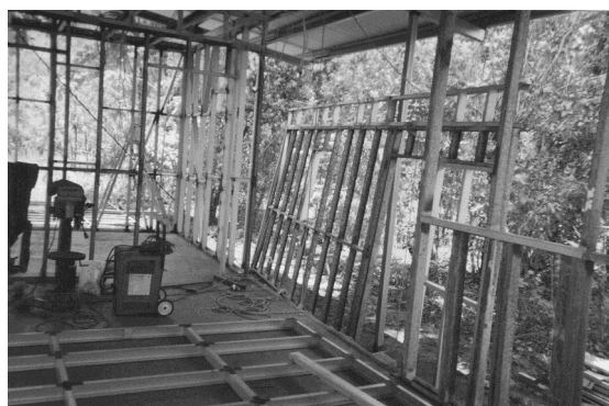
Wall frames, steel cutting and welding equipment
